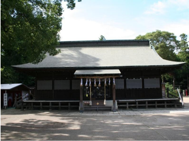
Figure 4: The Main Building at Washinomiya Shrine (2009)
