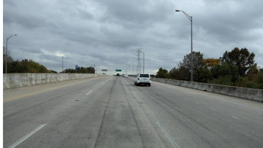
(f) Bridge Deck from TN-SR385
