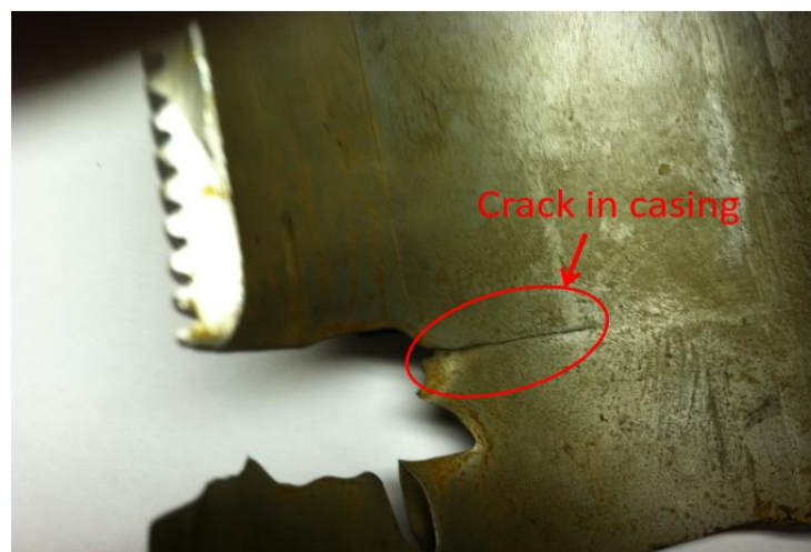
Figure 16. Crack in casing at last engaged thread of the frack head (Magill, 2013)
