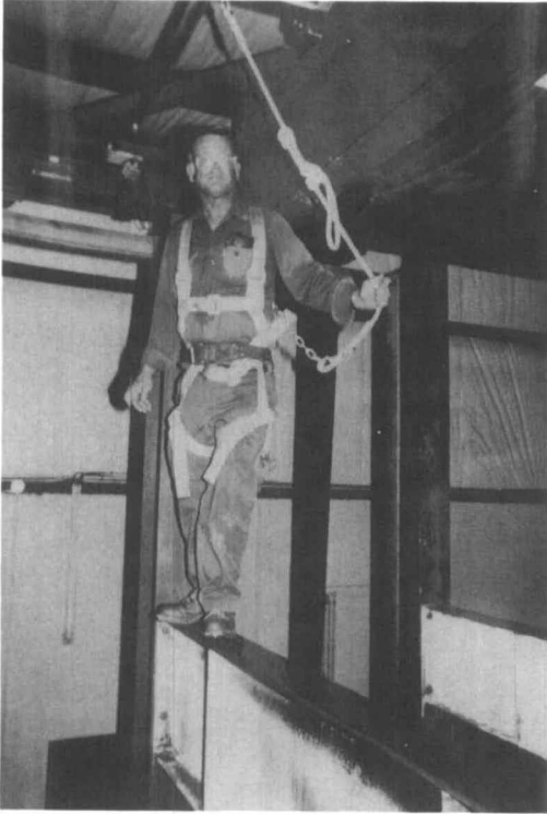
Figure 2. Ironworker with safety harness walking across a beam.
