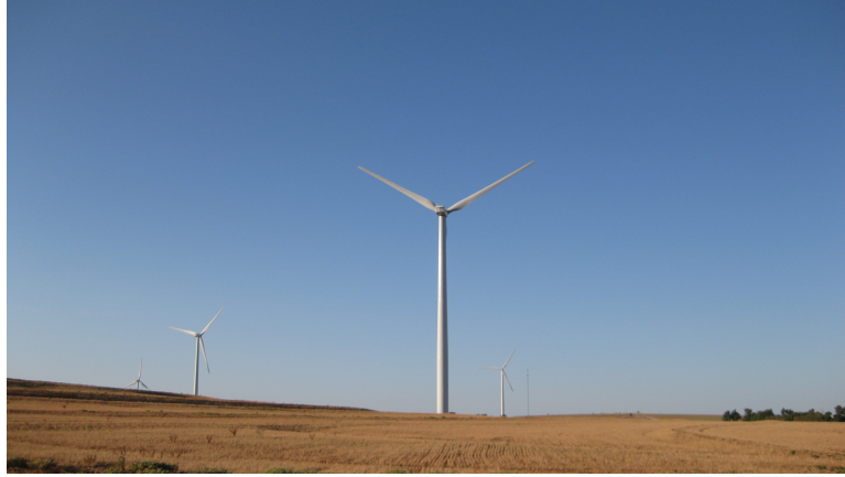
Figure 1.13: The state-of-the-art horizontal axis wind turbine manufactured by General Electric Company with a capacity of 1.6 MW. The wind turbine in the photo is installed near Minco, OK.
