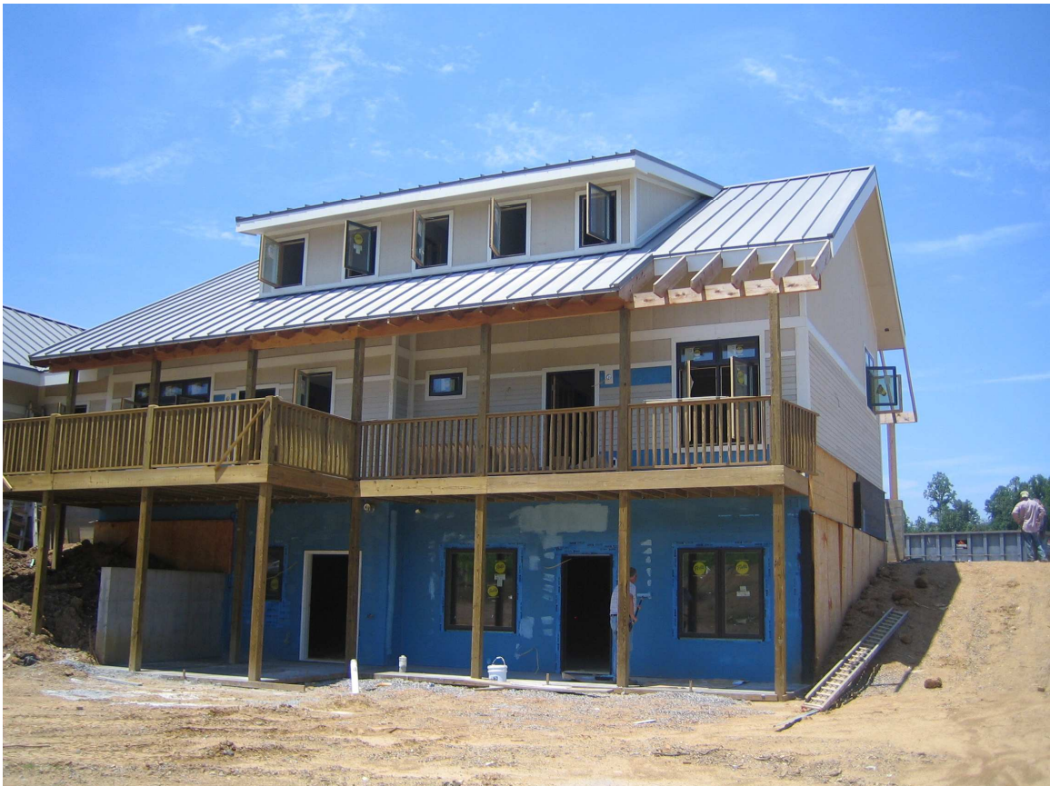
Figure 6.5: Experimental house built in Oak Ridge, Tennessee
