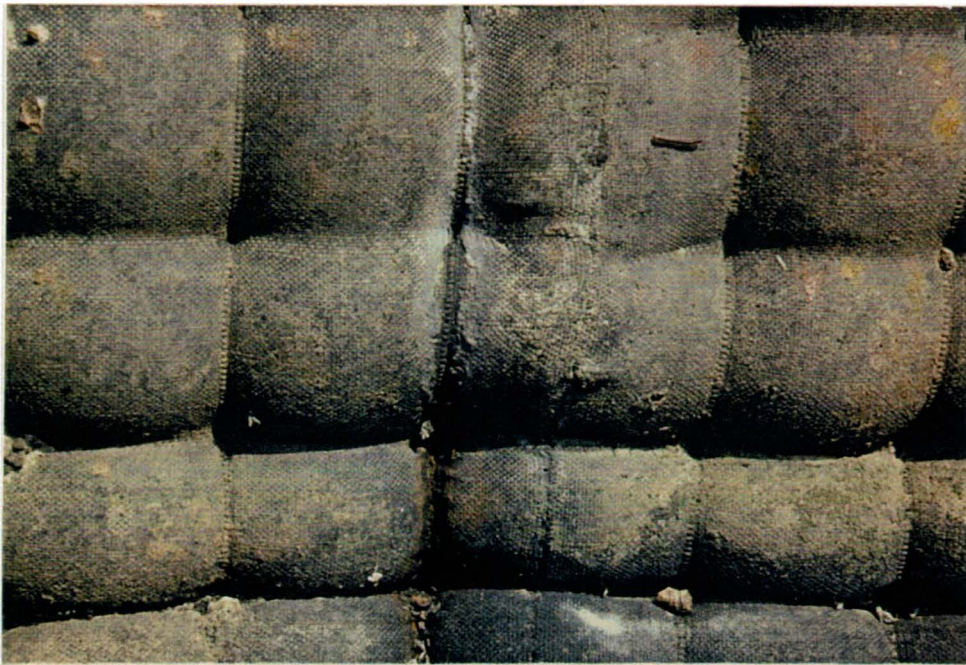
Illustration 10 Showing Bond (Nylon type)
