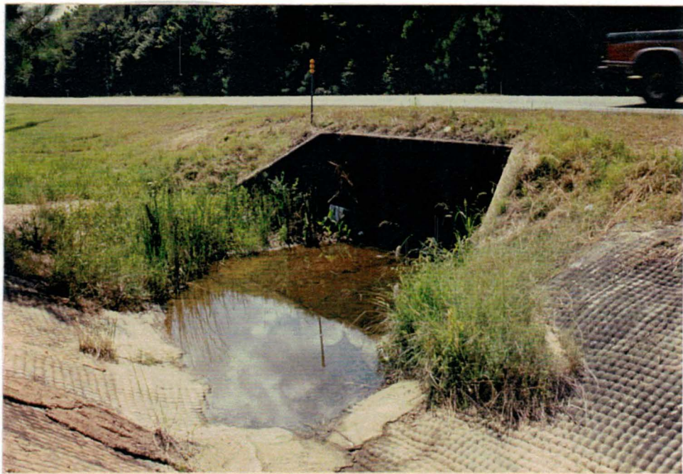
Illustration 2 Culvert at south end of ditch
