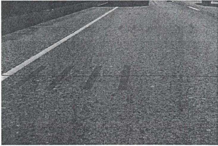
Figure 46. A completed load restoration project.
