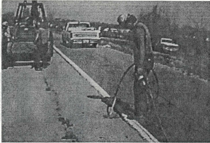
Figure 26. Vibratory compaction of repair material.
