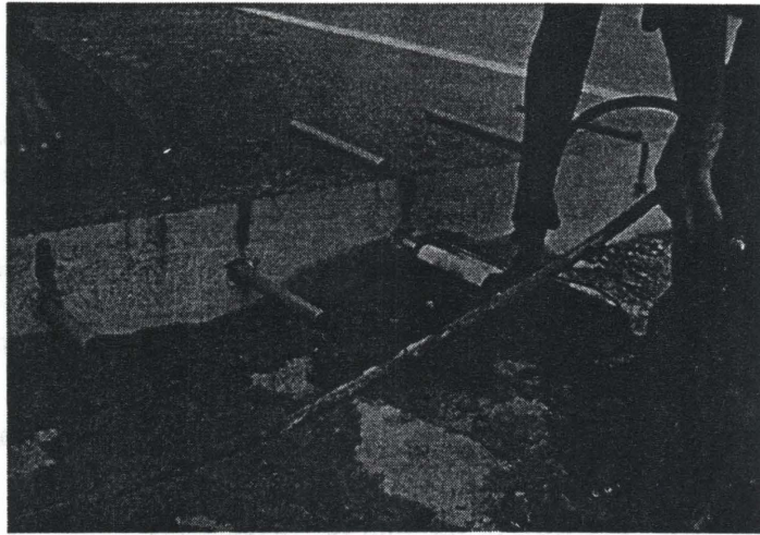
Figure 12. Epoxy resin injection into dowel holes.
