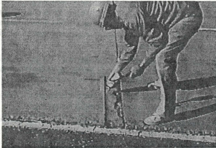
Figure 19. Marking of repair area.
